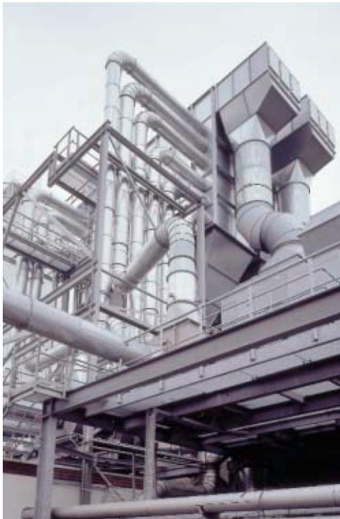
Amplly sized explosion vents in the return air ducts and an 180 degree bend prevent the pressure wave being propagated in the workshop.
