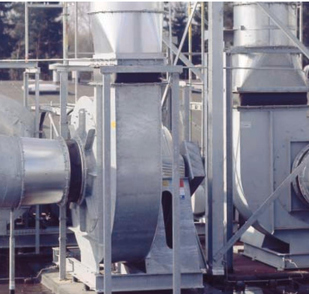
Fans which are continually exposed to extreme weather conditions or which operate in a humid medium can be provided with a hot-galvanised corrosion protection. We use fans made from rust-proof or acid-resistant steel for chemically aggressive media.
